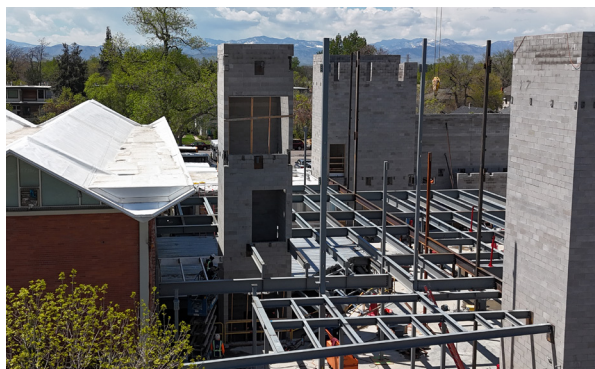
✨ Going vertical and steel placement
